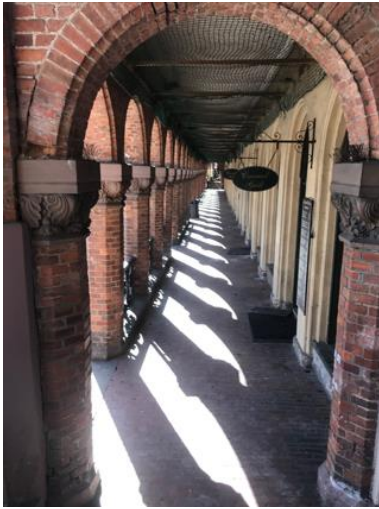
Figur 27 Ytre buegang langs Dronningens gate.
